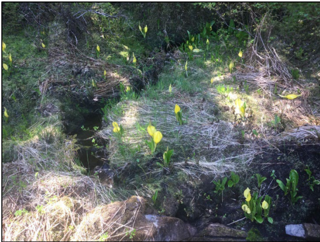
Figure 2.—Channel downstream of culvert outlet at waypoint 68.
